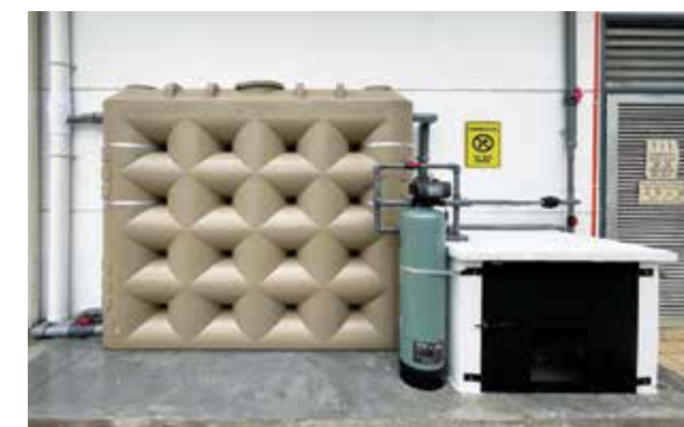
Rainwater harvesting system installed at PETRONAS station
